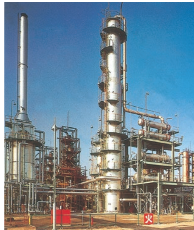
Petrochemical plant (304, 316L, S31803, e.t.c.)
